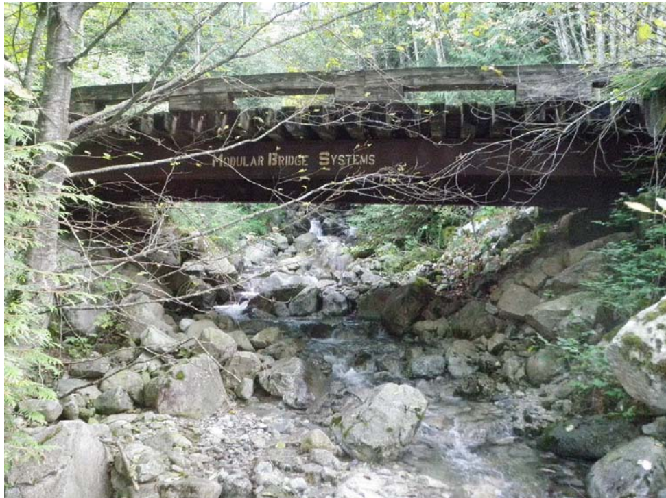
View from downstream
